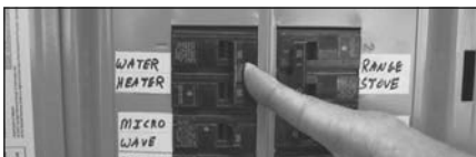
Figure 31 - Circuit Breaker
