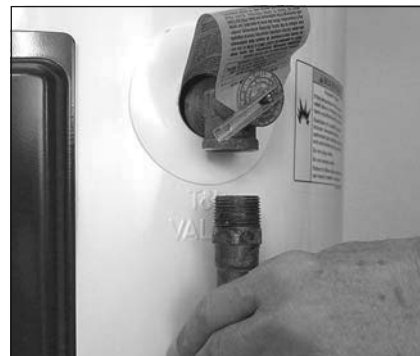
Figure 13 - Removing the T&P Relief Valve discharge pipe.
