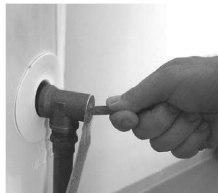
Figure 46 - T&P Relief Valve
