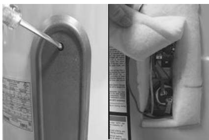
Figure 45 - Element Access Panel/ECO Compartment
