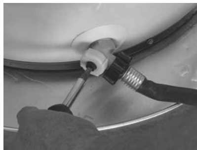
Figure 12 - Draining the old water heater.
