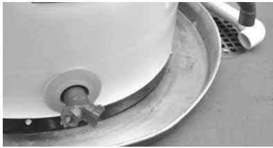
Figure 8 - A suitable drain pan piped to an adequate drain can help protect flooring from leaks and drips.
